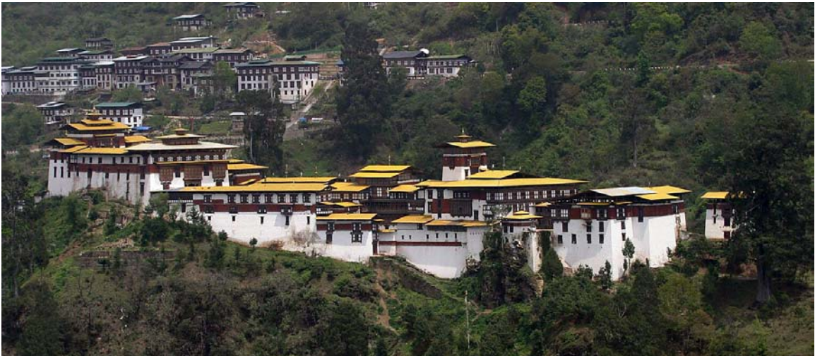
Trongsa Dzong, the largest Dzong in the country and long the seat of power. Dzongs combine a Buddhist monastery and a government administration center. They were built as fortified centers of power to govern the districts of Bhutan, which are formed from the four major river valleys of the country. Trongsa, Bhutan.
